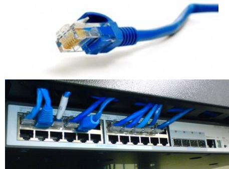
Figure 6 Ethernet Cat5 cable and switch
